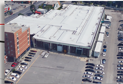
Danforth TTC Garage 1627 Danforth Ave
